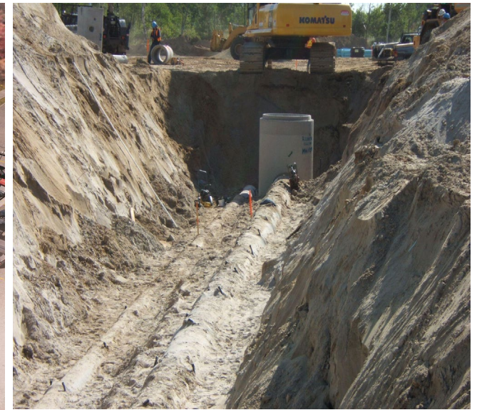
@Source-Energy™ Pipe Subdivision installation Sudbury, Ontario, Canada
