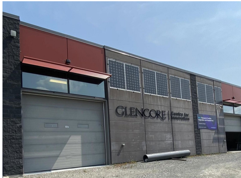
@Source-Energy™ Pipe and Panel Gold LEED certified Cambrian College Sudbury, Ontario, Canada
