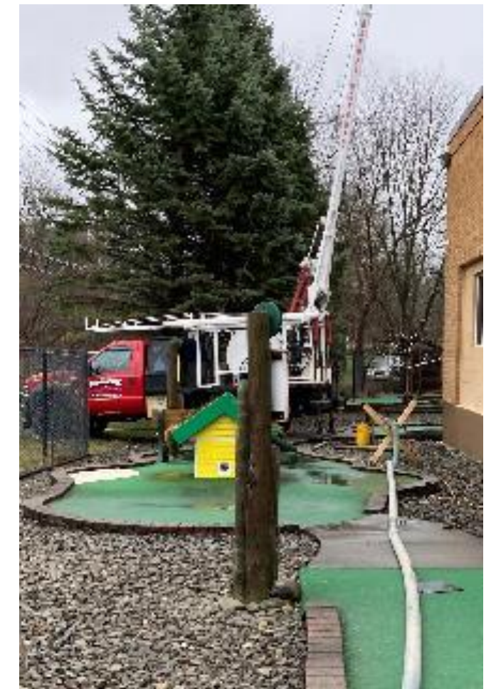
Image 6: 24 Hour Pump Test
