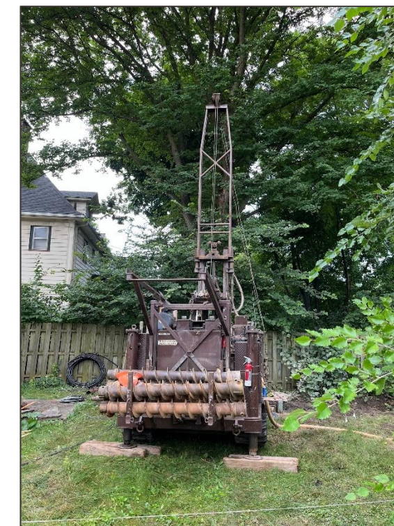
Image 9: Geothermal Drilling for Residential Home
