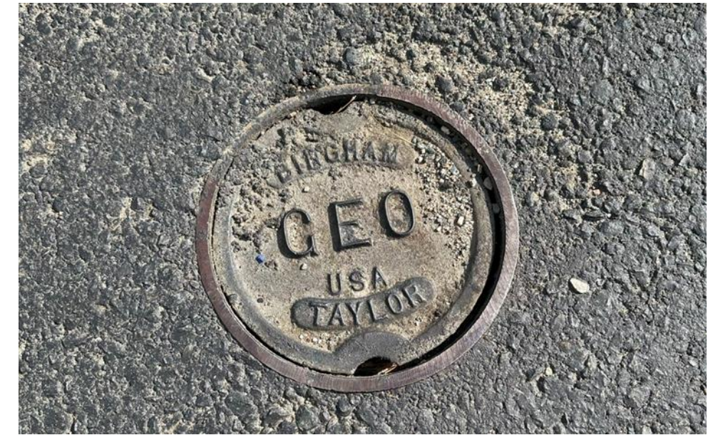
Image 7: Geothermal Handhole - Eversource
