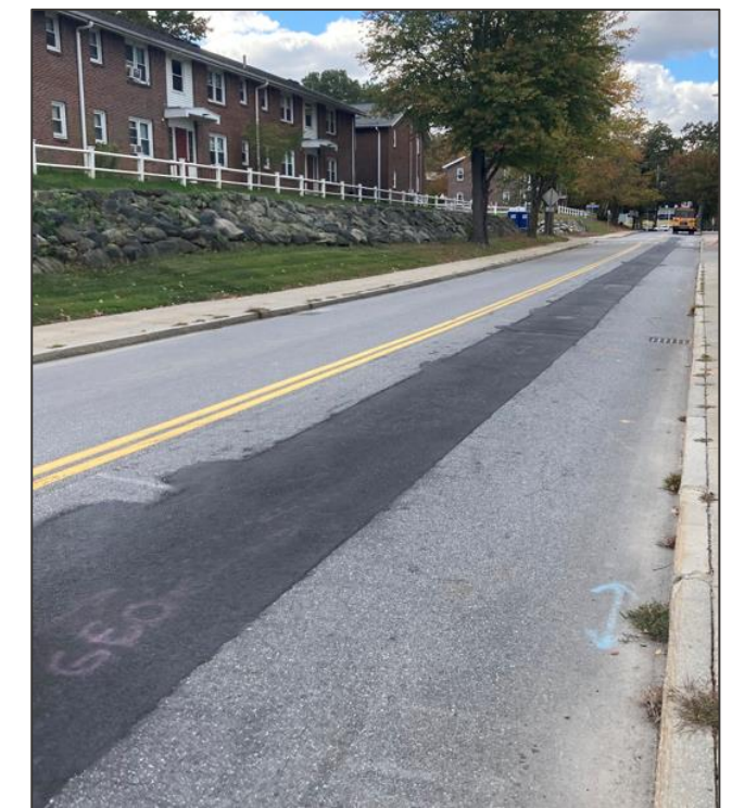
Image 10: Eversource - Thermal Distribution Main
