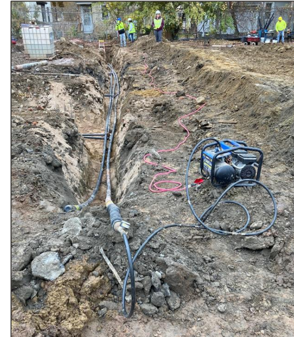
Image 6: Geothermal Header Pressure Testing – Customer System
