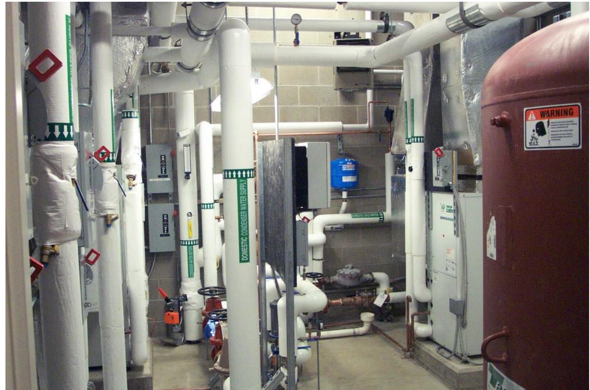
GHP system at NOAA's Caribou Weather Forecast Office in Maine. Photo courtesy John Porter / NREL pix 12708.
