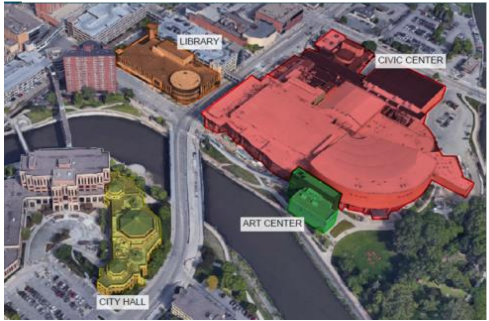
Rochester, MN city buildings that will initially be served by the geothermal district energy system. Rendering from Minnesota House of Representatives .
