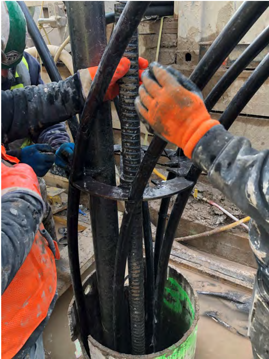
Loops equally spaced around circumference
