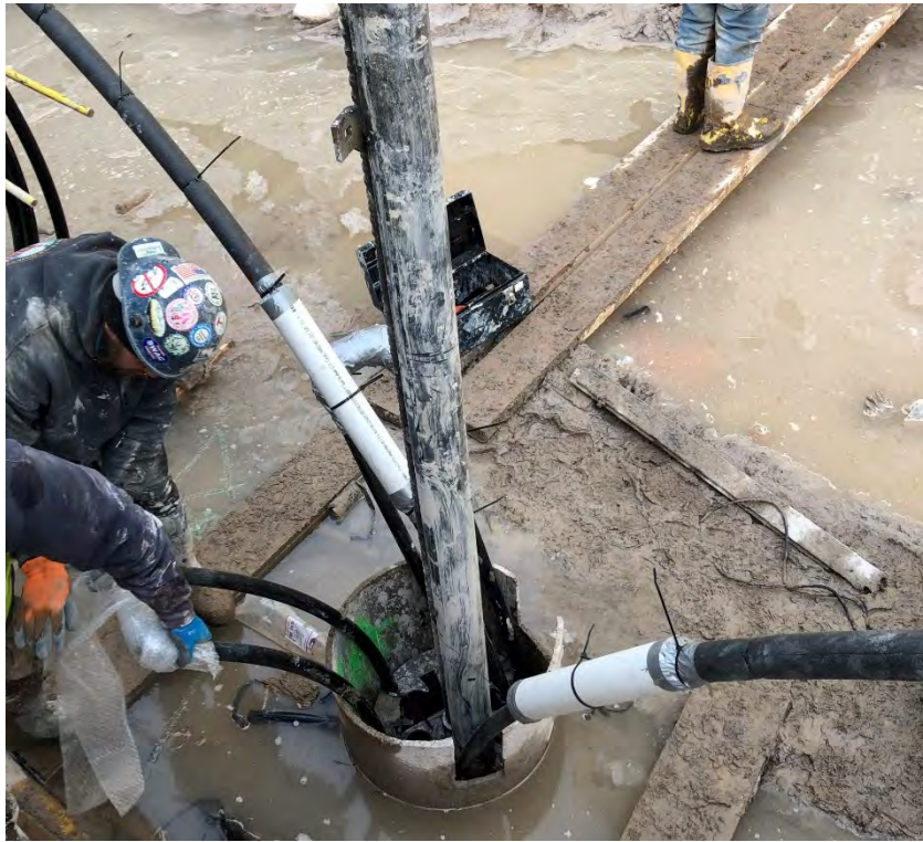
QA/QC Flow & Pressure test
