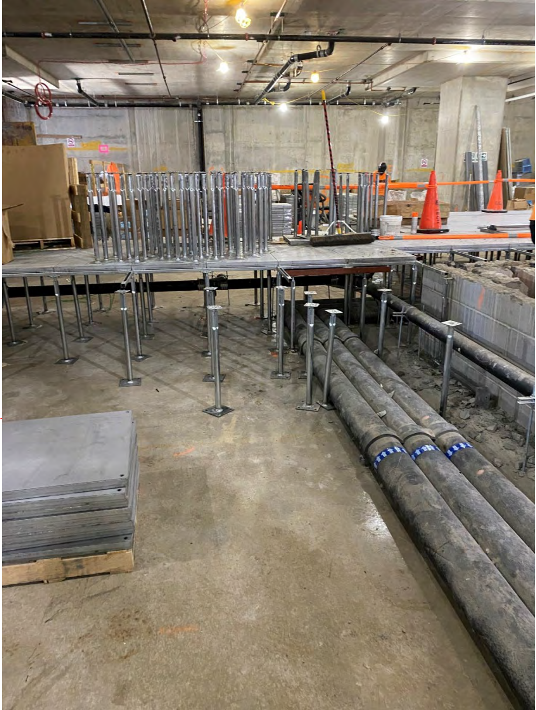
Removable flooring being installed
