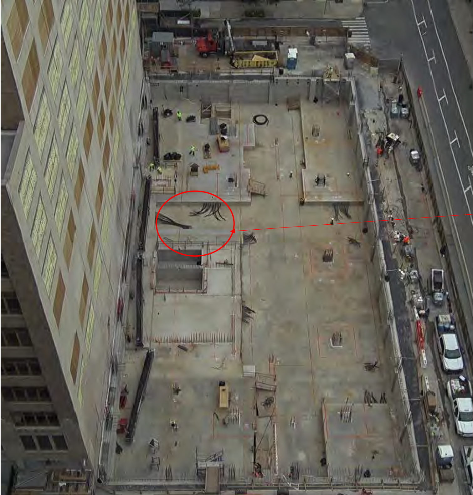
Each geo loop fitted with pressure gauges to verify system until next stage
