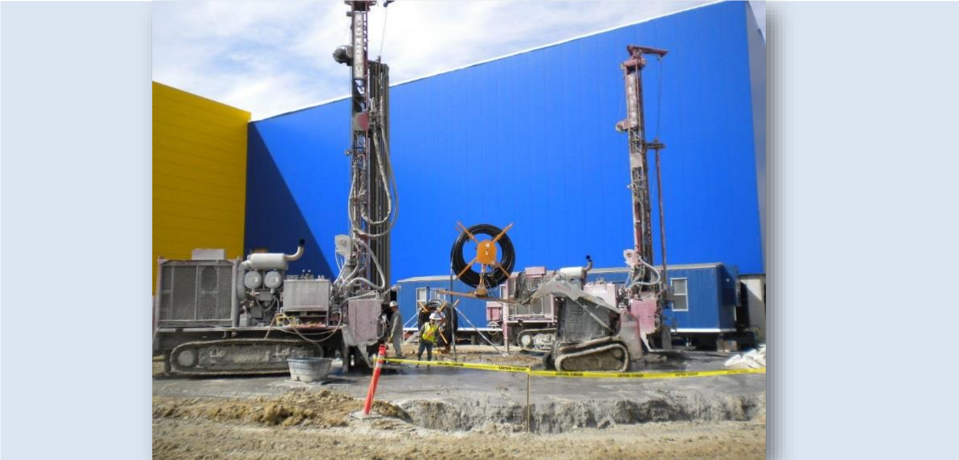
600' depth loop installation in progress
