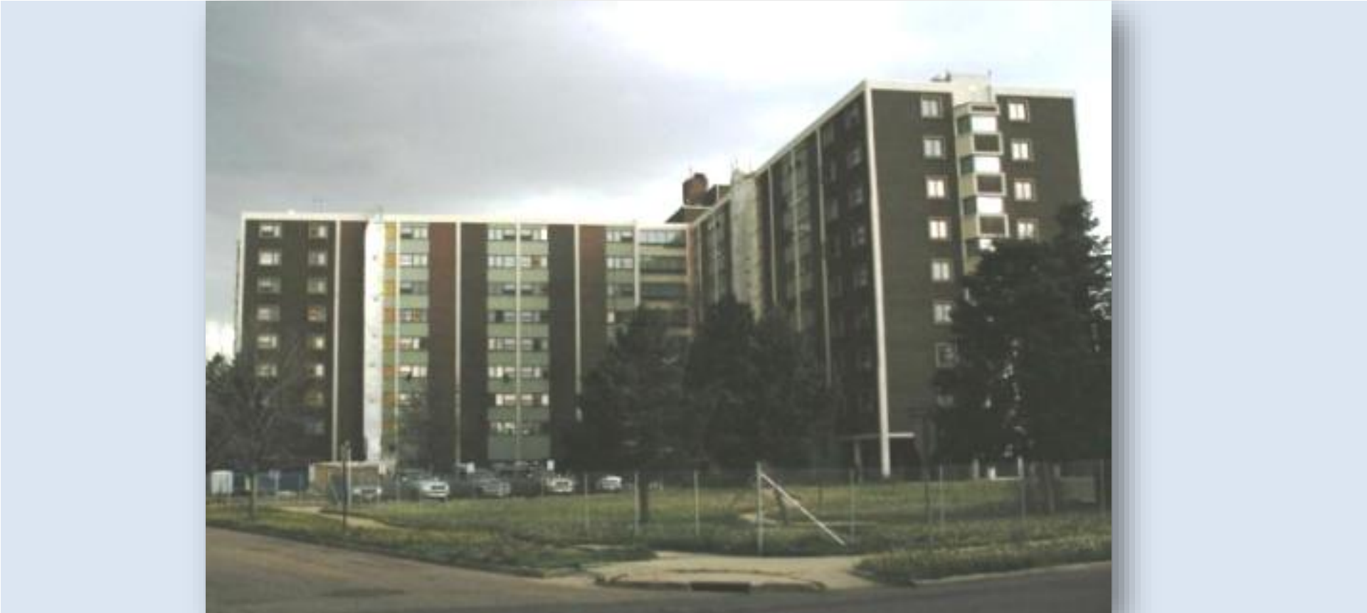
81 boreholes x 450' depth x 1.25" DR11 Nine story facility (Hirschfeld Towers, Denver, CO)
